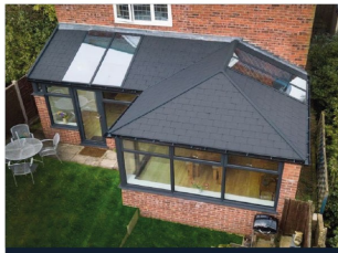
Replacement Tiled Roof
