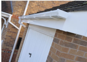
Fascia Soffits & Guttering
