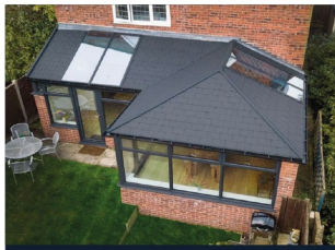
Replacement Tiled Roof
