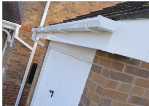
Fascia Soffits & Guttering
